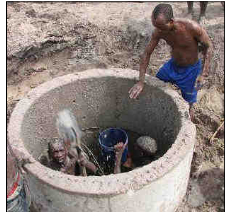
Two men in the well, one digging and the other bucketing out water.
